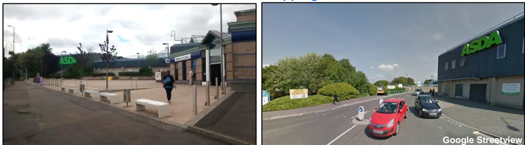
Front and Back Entrances to The Avenue shopping centre
