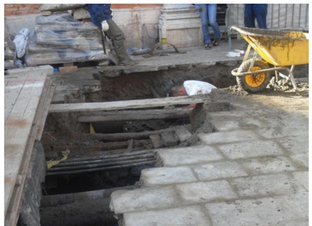
The key driver should be that all services are provided such that they can be maintained without damaging or affecting the road design life. Ducting is considered an acceptable method of providing denser utility provision which permits upgrades without extensive road disruption.
